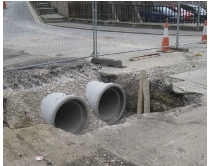
Drainage New Beck Hill 2017/09/07 15:11
