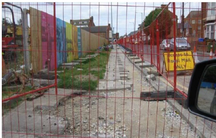
Before New Beck Hill Bridge 03/02/2016 13:59
