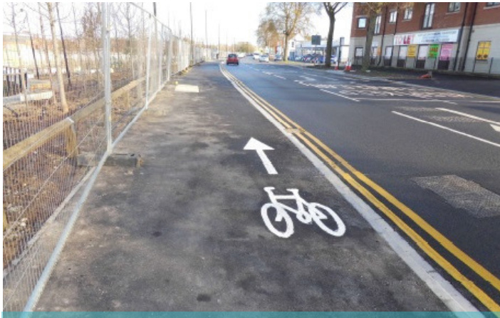
Shared use cycleway Hilderthorpe Road 2019/02/11 13:25
