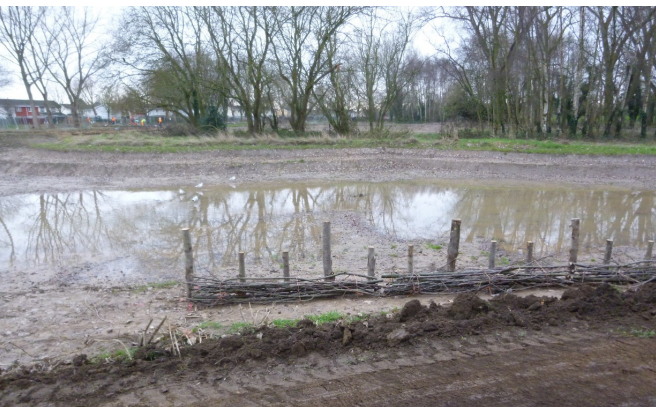
COPFAS - Phase 1 Fishing Pond banks under construction 12:22 10/JAN/2019
