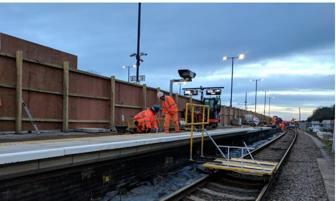
Works at Barnetby Station (3)
