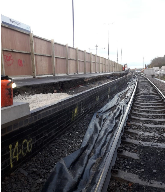
Works at Barnetby Station (2)
