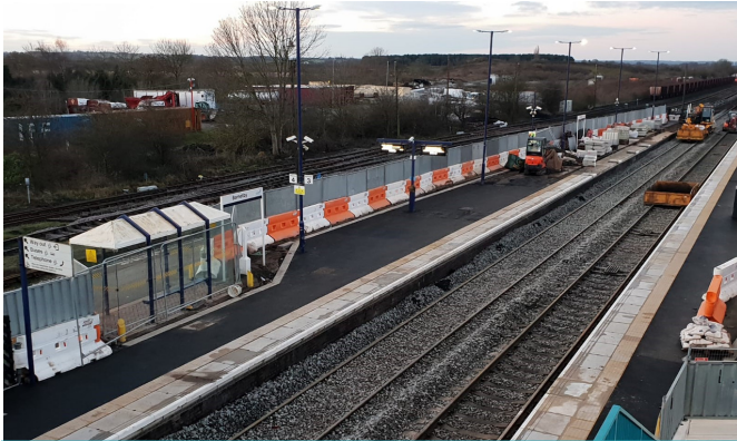
Works at Barnetby Station (4)
