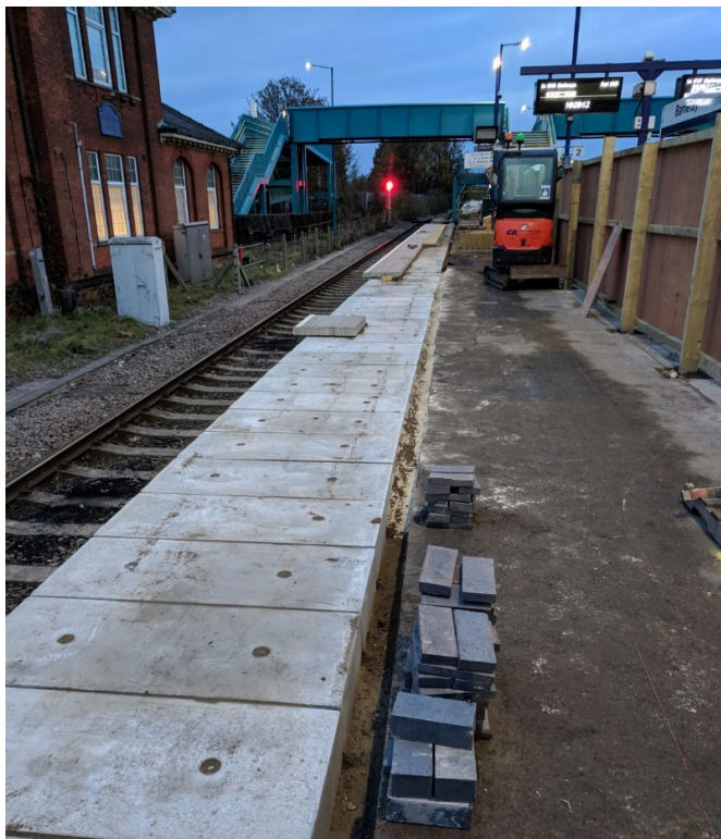
Works at Barnetby Station (1)
