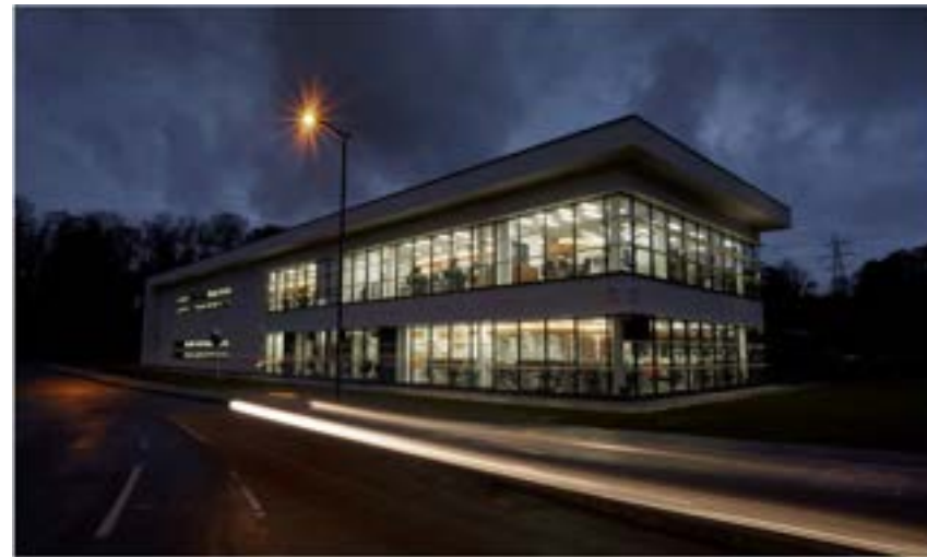
Woodland House Offices, Hesse
