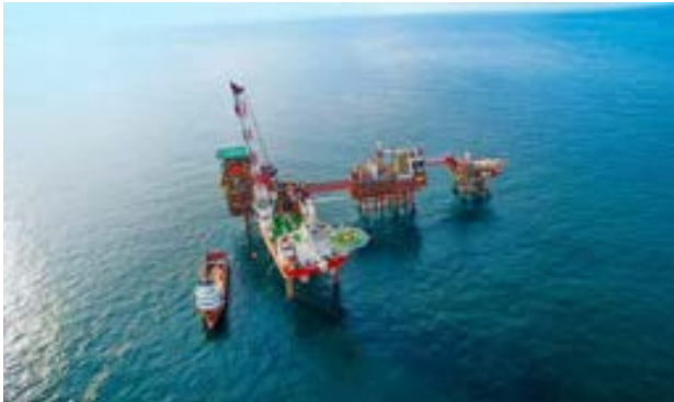
47/3B Offshore Platform ~30km off the Easington coast
