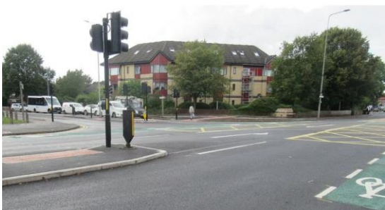
A view of the new look pedestrian crossing.
